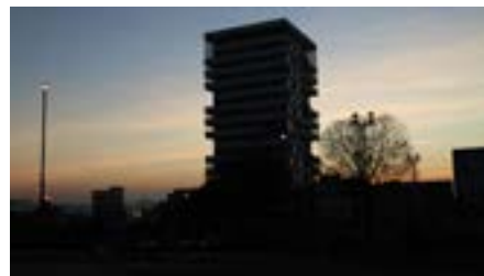
This Barcelona doesn't appear in the postcards. The panoramic taken from Torre Júlia allows comparing the building with the urbanism around: This architecture is a representation of the 'banlieue' architecture from the 60's and 80's.
